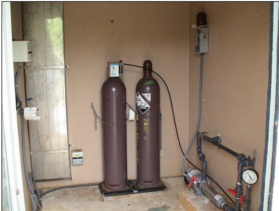
Figure 1-5 – Typical Indoor Well Chlorination System Installation
