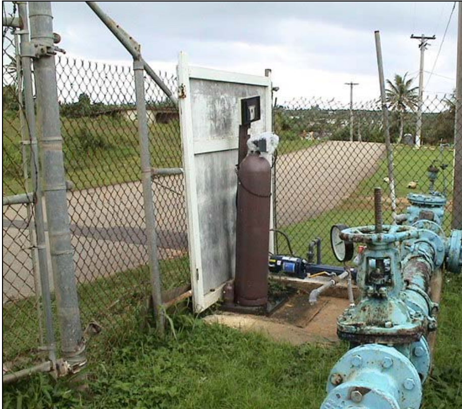
Figure 1-6 – Typical Outdoor Well Chlorination System Installation
